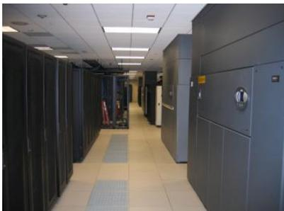
Data centres located across the globe have been simulated, involving complex single-or-multi-room layouts, under-floor ventilation, sometimes a return air ceiling plenum and cold aisle containment systems. CHAM personnel and agents have performed site surveys, gathering detailed information on the layouts and cooling systems, which, together with engineering drawings, enabled 3-D models to be built using CHAM's streamlined method.
