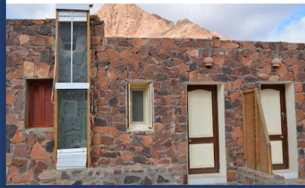
Figure 2. The Trombe wall ventilation system (left) has been modified to be used both for heating and cooling using renewable energy sources. Researched by Marwa Dabaieh from Lund University in Sweden. Tested in Saint Catherine, Egypt Photo: Insaf Ben Othm
