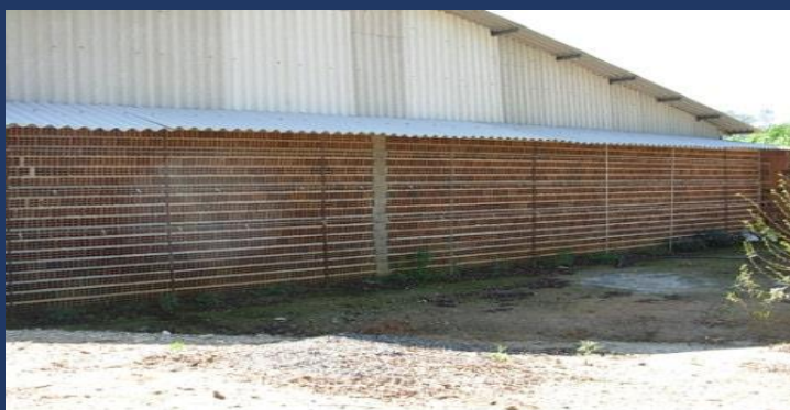
Figure 2 Porous wall (inlet)
