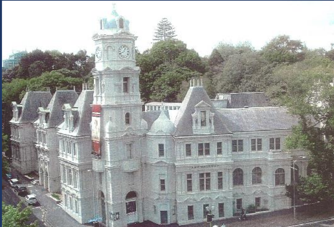
Existing structure Auckland Art Gallery
