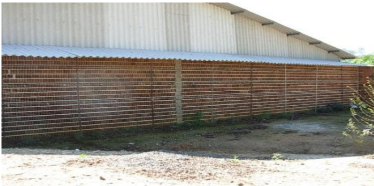
Figure 2 Porous wall (inlet)
