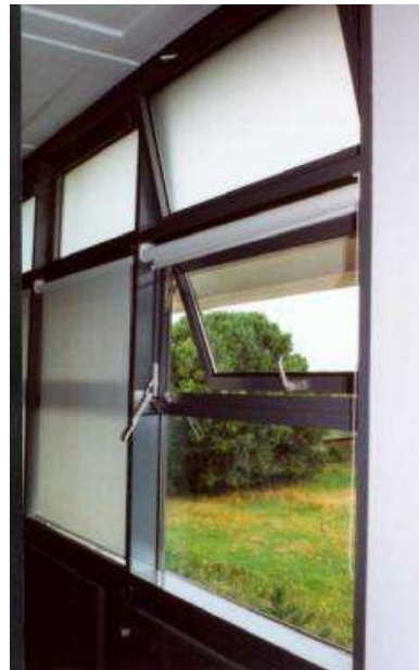
Figure 6. Interior View of Window
