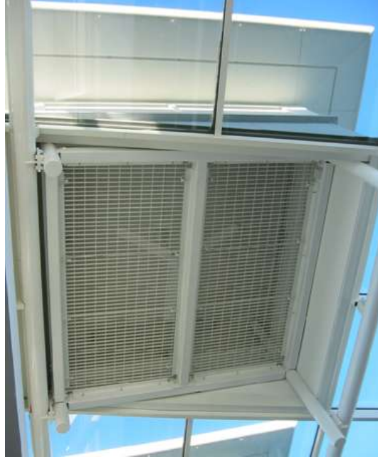
Figure 13. Atrium Stack Vent and Fan
