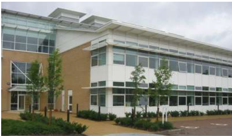
Figure 14. Exterior View of Southern Facade of Prototype Building
