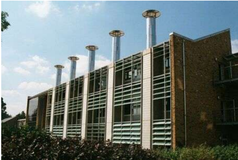
Figure 1. BRE Office Building Facade with Stacks 1
