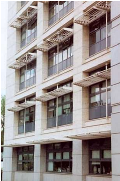
Figure 5. Edinburgh Gate Office Building Exterior Facade
