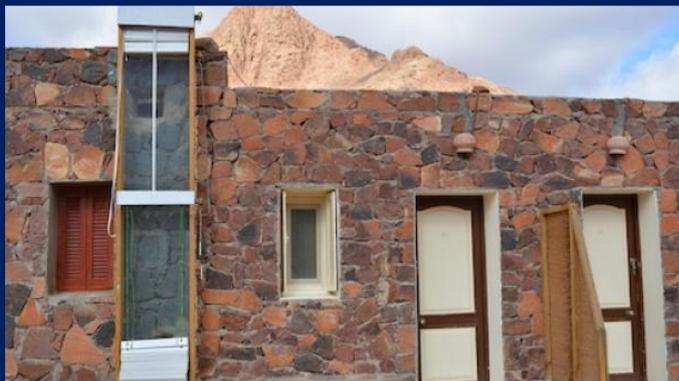
Figure 2 The Trombe wall ventilation system (left) has been modified to be used both for heating and cooling using renewable energy sources. Researched by Marwa Dabaieh from Lund University in Sweden. Tested in Saint Catherine, Egypt Photo: Insaf Ben Othman
